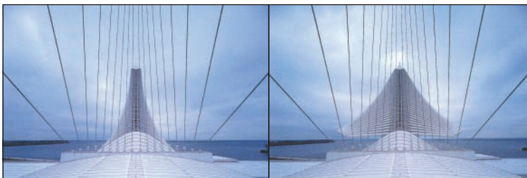
Plate 7: A timed view showing the movement of the building. The winged structure opens and closes with the museum's visiting hours.
