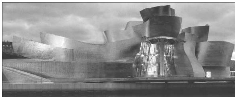
Photo of final building
